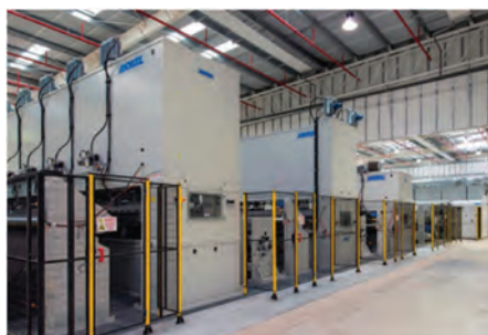
Industrial production line located ANDRITZ Asselin-Thibeau
